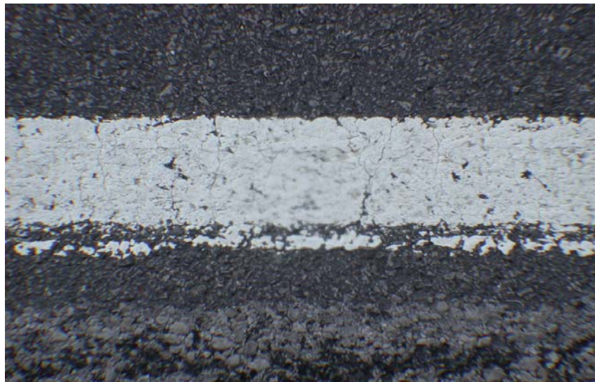
Figure 3-2. Flat thermoplastic marking
